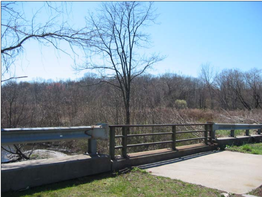
SOUTHWESTERLY VIEW OF PENINSULA FROM SPILLWAY ON BOWMAN AVENUE
